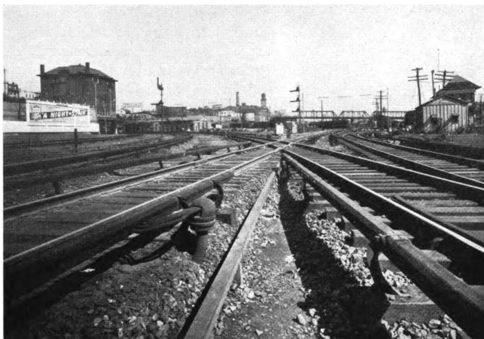
View of Right-of-way Showing Third Rail
