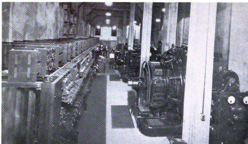
Substation No. 1B at 43rd Street. 2000-kw. Synchronous Converters
